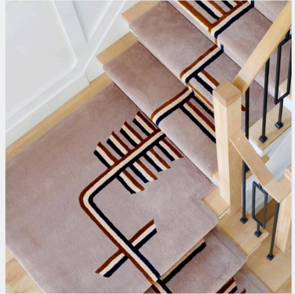
Custom "Health" staircase installation
